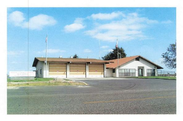
Station 82 was built in 1986 and is a single story, 5,829 square foot wood frame with stucco exterior siding and a composition shingle roof.
