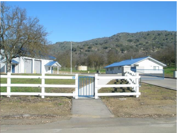
Current Sand Creek Station
