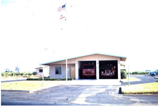
Station 20 in the early 1960's
