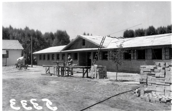
inmate barracks construction 1954
