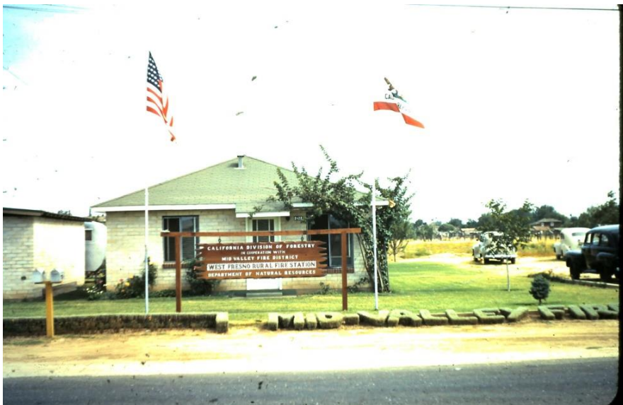
West Fresno Station (note hedge pruned to show Mid Valley Fire, spelled out)
