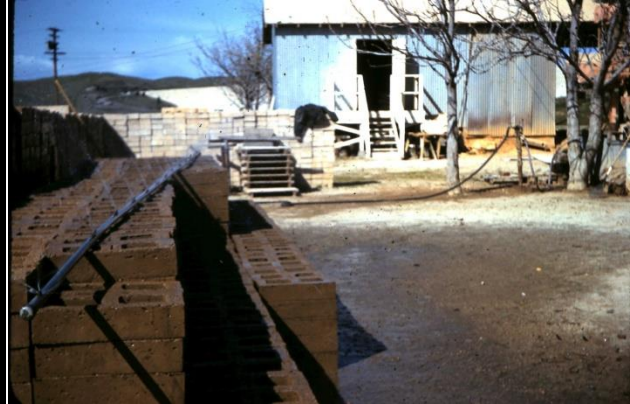
Curing the brick following manufacture
