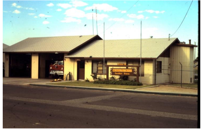
Station 10 after the additional bay was added.
