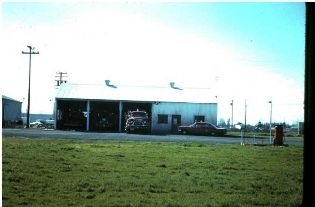
First Station 7 with 3 apparatus bays
