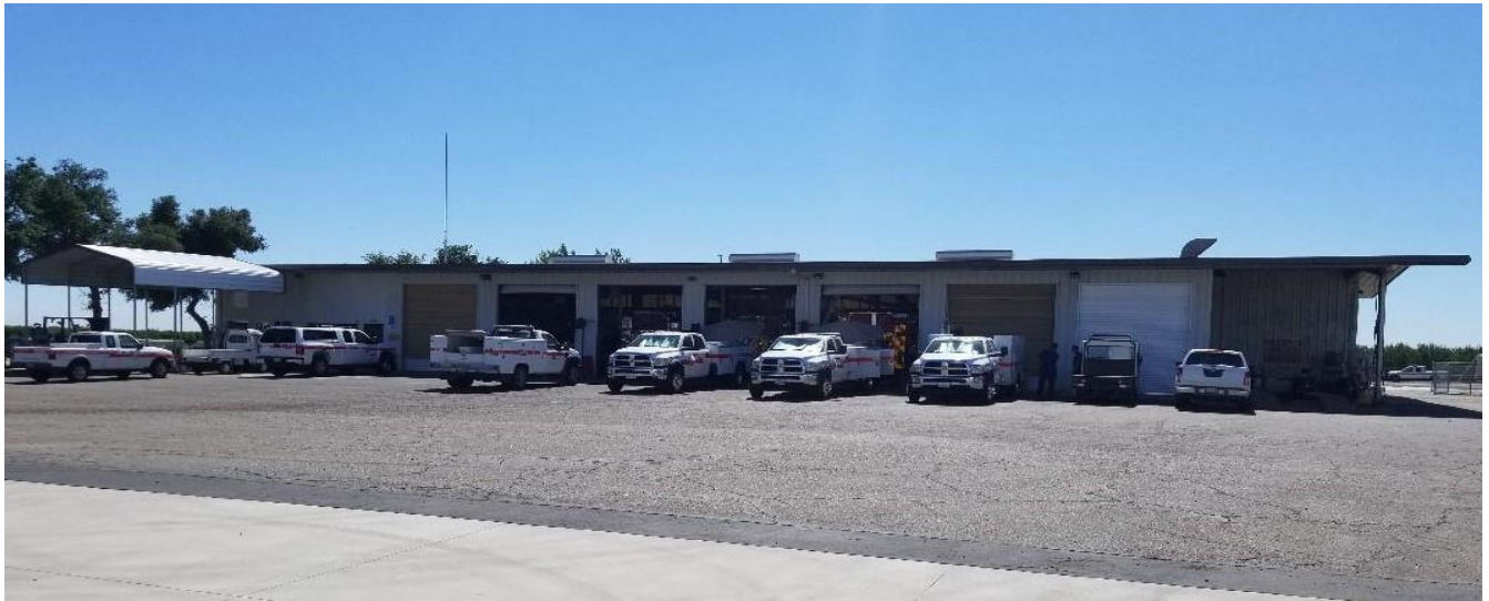
Current shop and offices @ Station 82
