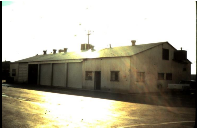
Station 7 after the addition of 2 bays & an office in 1967
