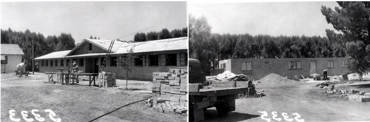
1954 construction of the inmate barracks and dining hall
