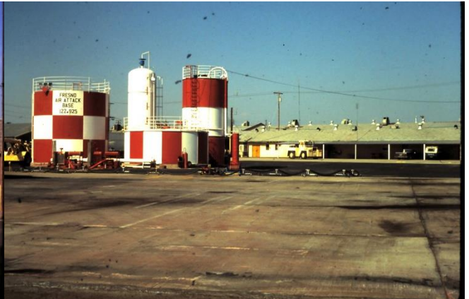
Old Batch plant and offices in the background
