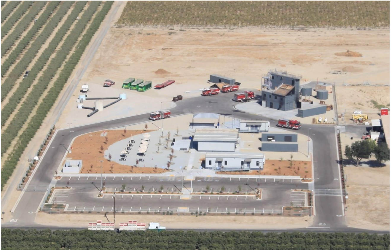
Aerial view of the training center
