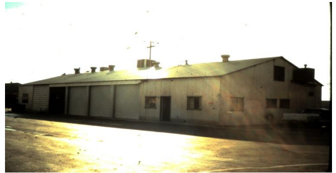
After addition of 2 bays & Office & parts storage
