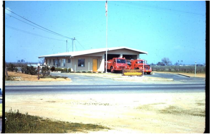
another view, note Herndon Ave as a 2 lane country road
