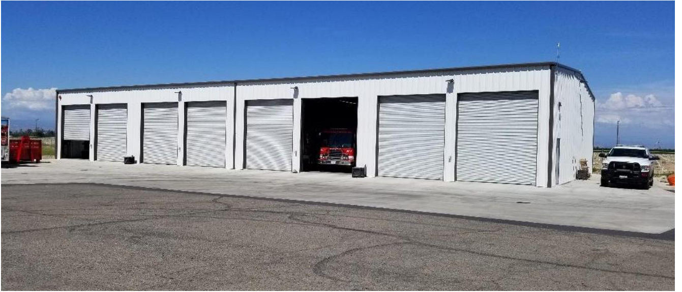
Reserve fleet storage building
