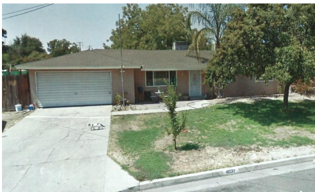
Tarpey Station (house) as it appears today
