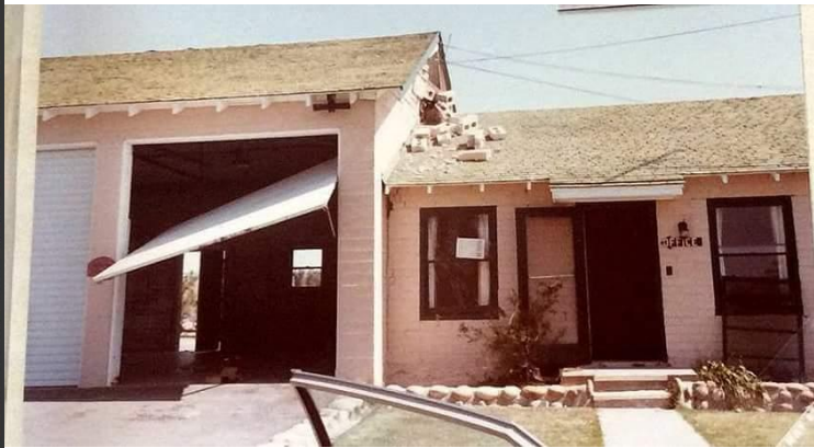
Oilfields Station following the earthquake.
