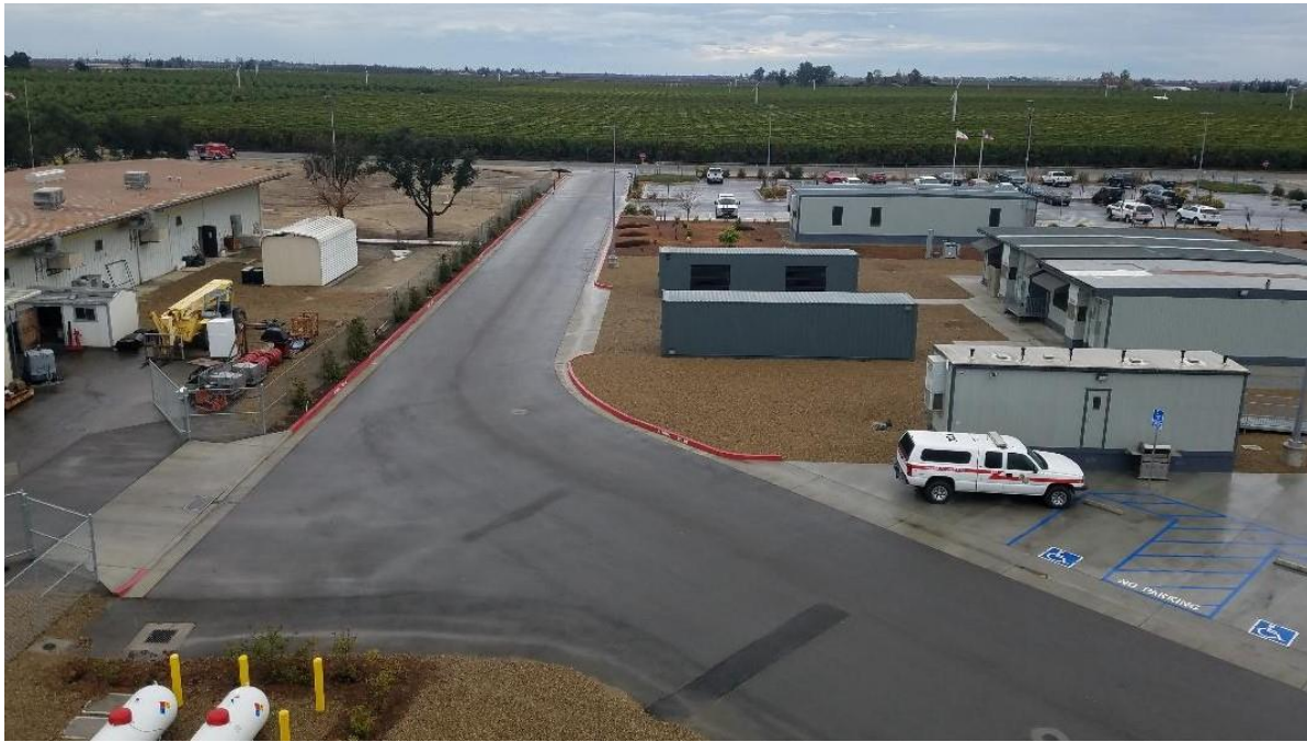
Classrooms, Offices on the right Back of the shop facility on the left
